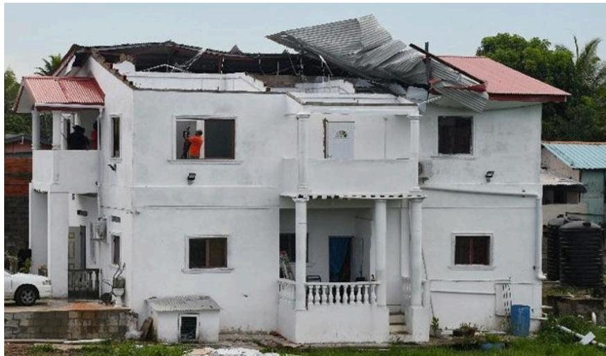
Across the Caribbean, roof failures have become an all-too-familiar sight after periods of strong wind. What makes this especially concerning is that many of these failures occur during moderate wind events, conditions well below hurricane strength.
